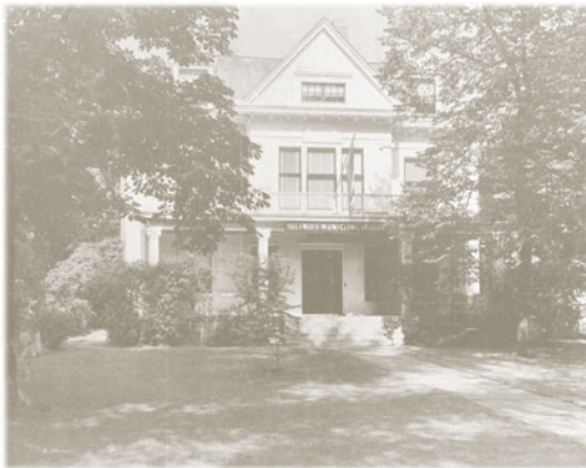
Broadwell Mansion – 1942 First Headquarters of the Association
